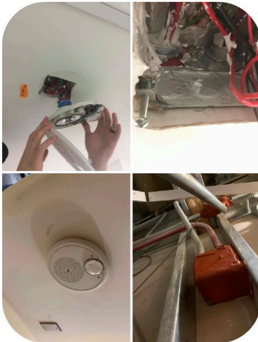
FIGURE 2. Example of photographs taken to document compliance with sealant requirements.
